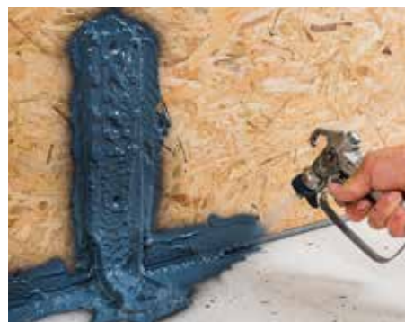
Airtight spraying over angle brackets,
