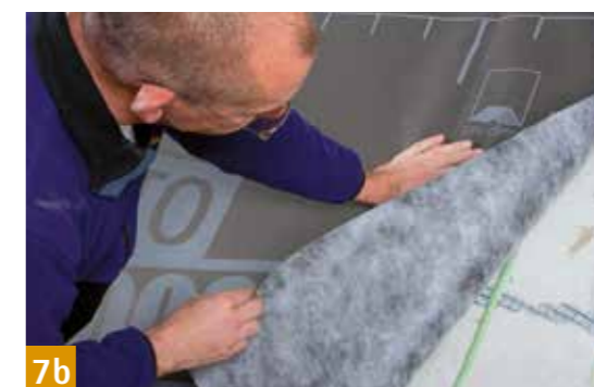
ORCON F Creates reliable joints with rough or mineral adjacent building components
